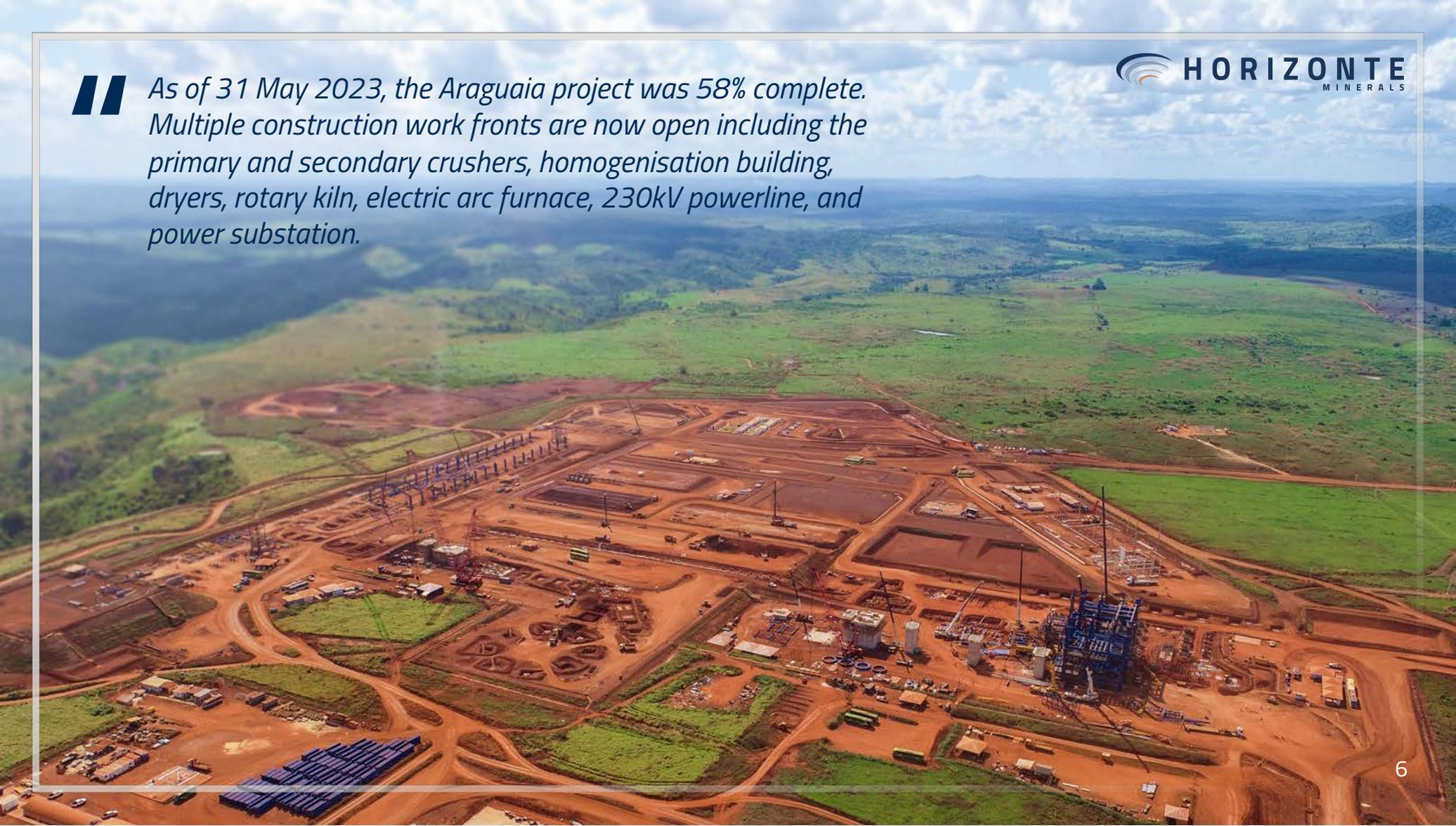
“ The electric arc furnace is manufactured by Hatch Ltd. At 18m diameter, the side walls and base plate of the furnace have been welded and the surrounding steel support structure that will house auxiliary equipment including the transformer, continues to be erected. The 4<sup>th</sup> of five floors is currently being installed.
