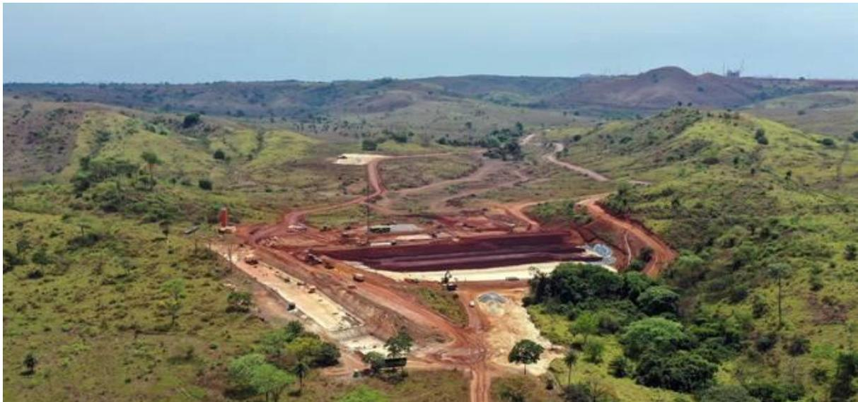
*Water Storage Reservoir where the Cofferdam is now completed and construction of the principal embankment is underway.*
