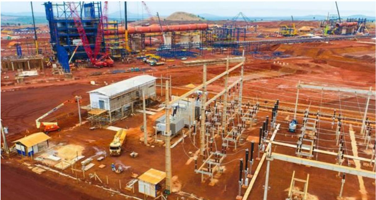
*The Araguaia sub-station with both of the main 230kV/34.5kV transformers installed.*
