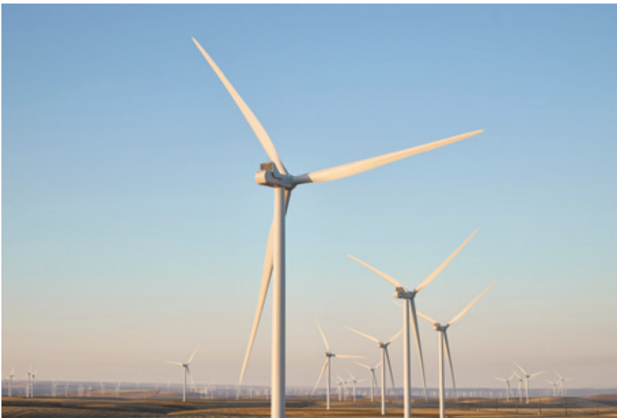
The Montague wind farm in Oregon is one of Apple's largest projects at 200 megawatts and powers Apple's Prineville data center.
