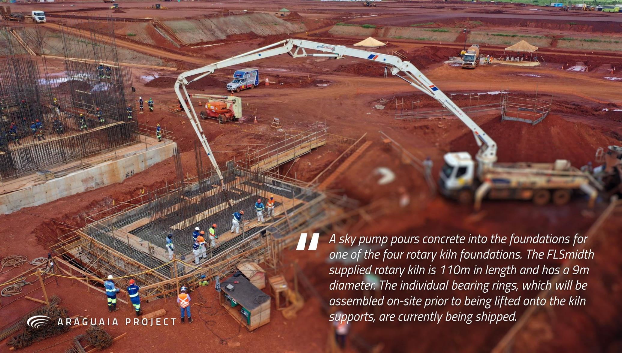
“ A sky pump pours concrete into the foundations for one of the four rotary kiln foundations. The FLSmidth supplied rotary kiln is 110m in length and has a 9m diameter. The individual bearing rings, which will be assembled on-site prior to being lifted onto the kiln supports, are currently being shipped.
